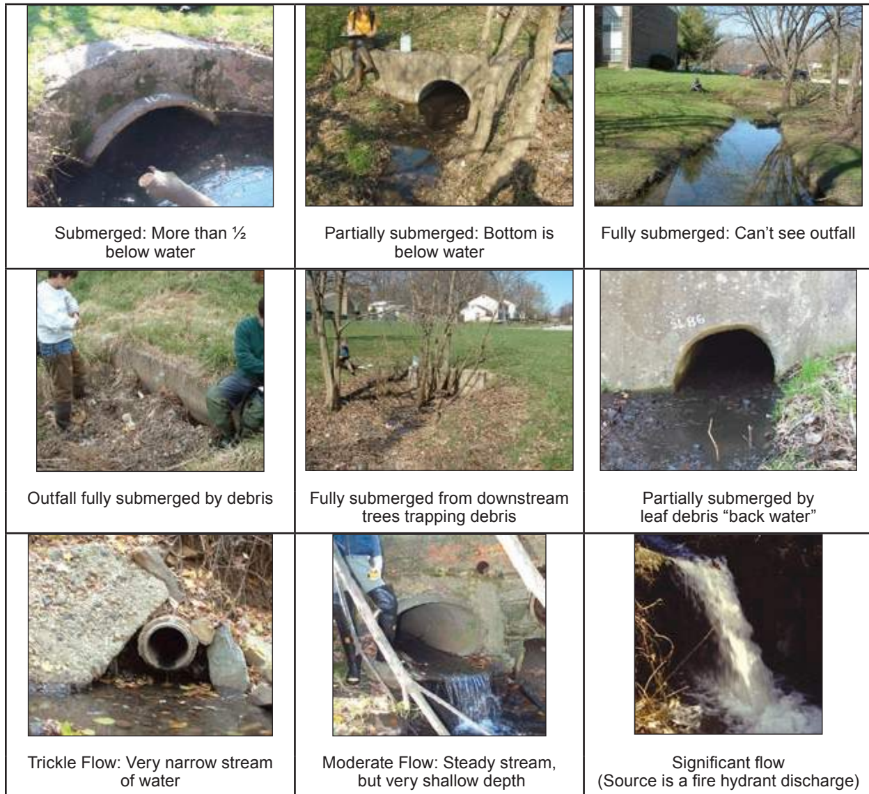
Figure 28: Characterizing Submersion and Flow
