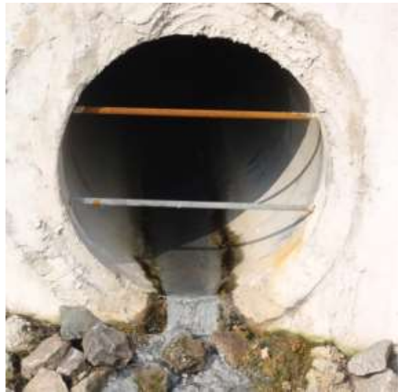
Figure 2. White/gray material seen in the pipes is a bacterial plaque often indicative of sanitary sewage.
