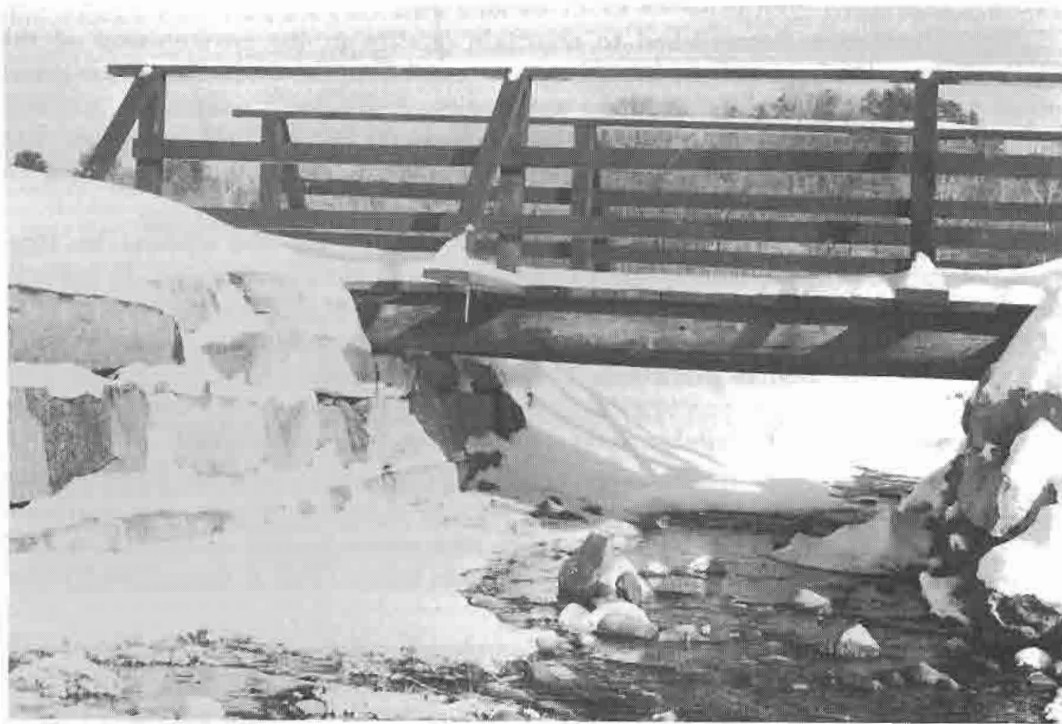
Recently Constructed Foot Bridge at Hampden Memorial Park
