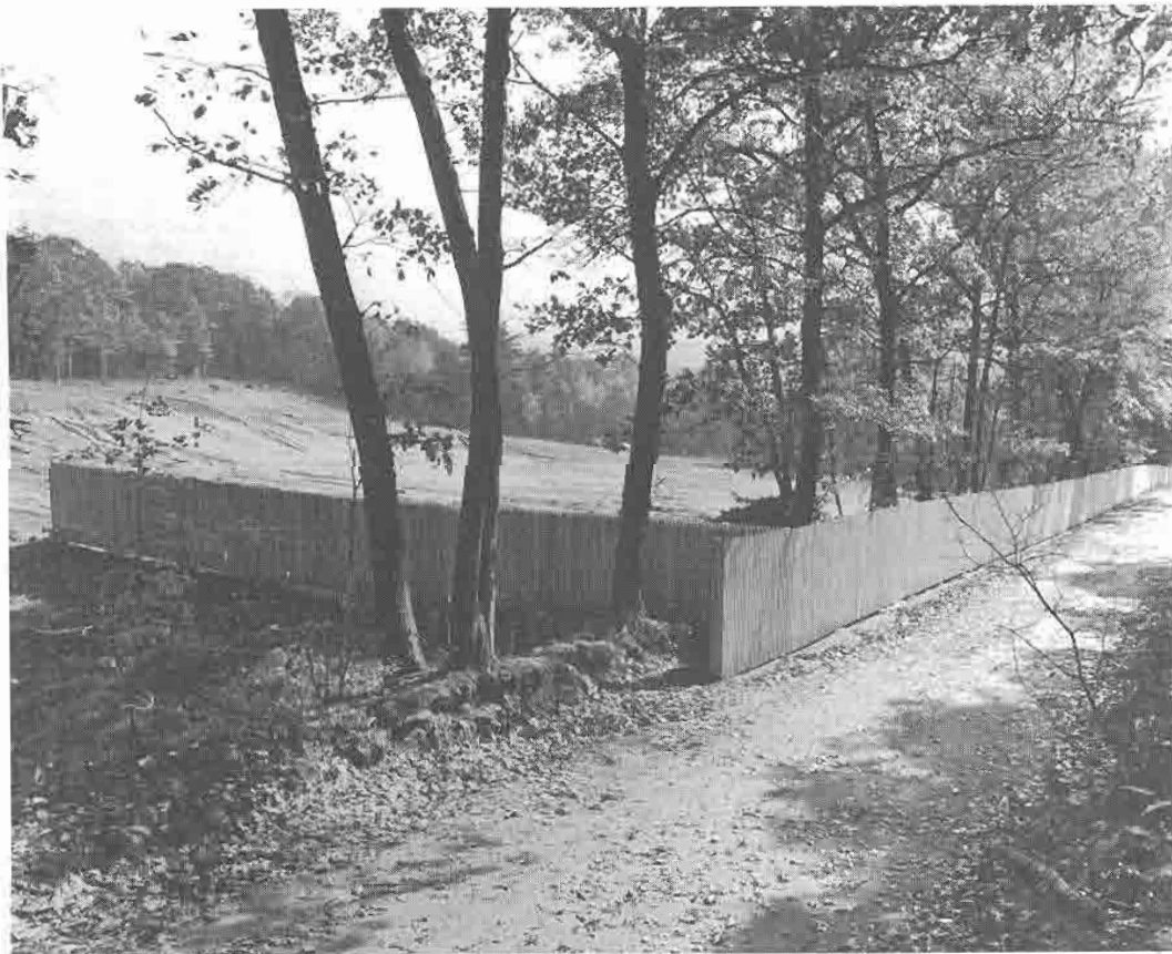
HAMPDEN SANITARY LANDFILL OPERATION —Graphic evidence of greatly improved conditions at site of former town dump.
